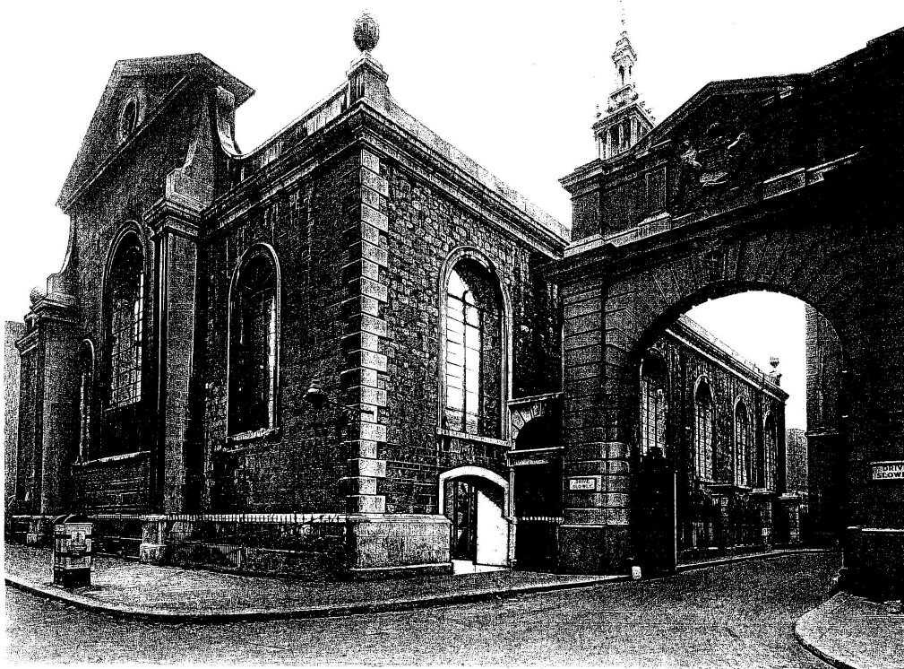
Christ Church from King Edward Street: the exterior as it appeared prior to demolition of the east and south walls. The picture uses a wartime photo, retouched to remove debris from the Blitz. The opening under the end window is added to show how the pedestrian route through the church site could be accommodated in a reconstruction.
