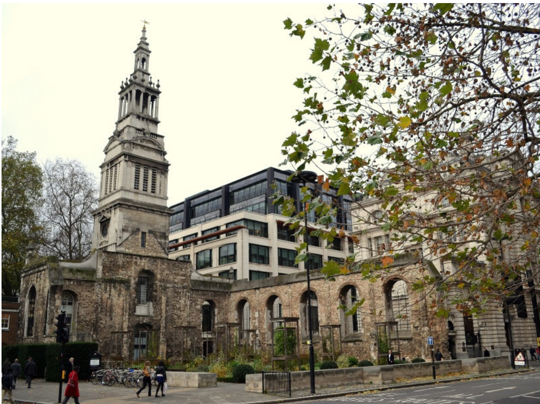
The Christ Church site seen from the BT Headquarters at the corner of Newgate Street and King Edward Street.
